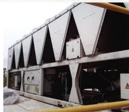
AHU & Chiller(Centralized Air-Conditioning)
