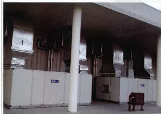
AHU & Chiller(Centralized Air-Conditioning)
